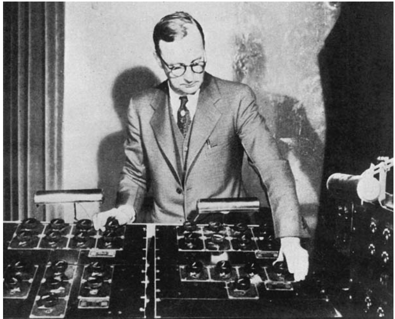
Master control system for all sound apparatus, located in a box on the 4th tier.
