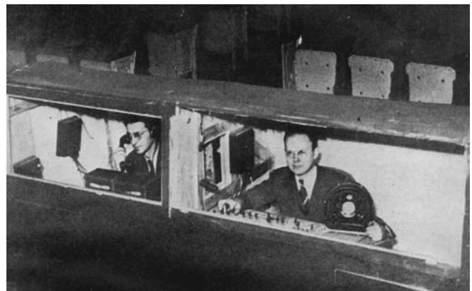
Dual prompters' box facing stage controlling sound and lights. Loud speakers become microphones at throw of switch.
